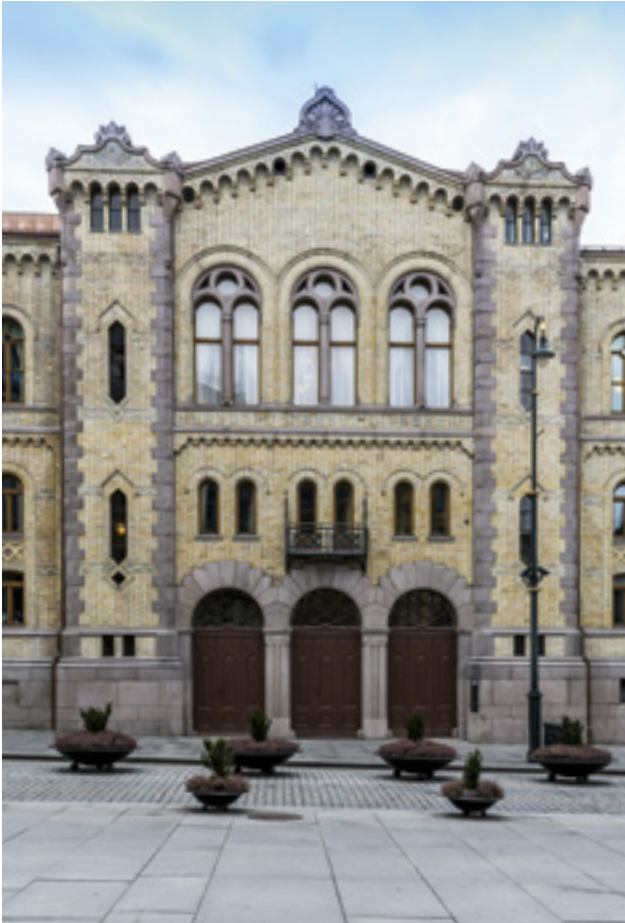
The protruding centre part of the façade facing out across Karl Johans gate marks the end of the cross-wings. The three doors are the public entrance to the Storting Chamber. (Photo: Hans Kristian Thorbjørnsen)
